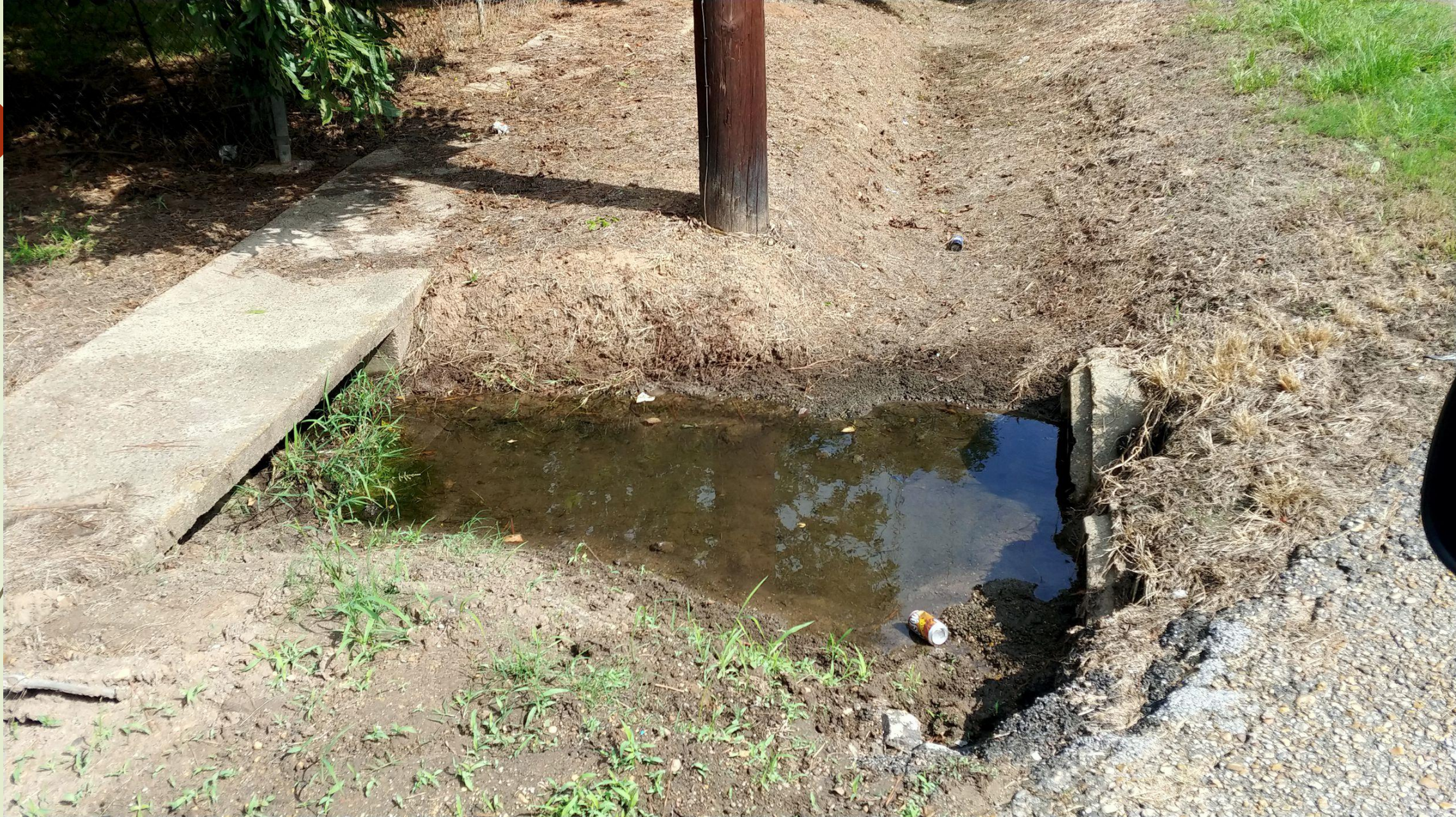
Culvert at the corner of Riverside Dr. and Norwood St.
