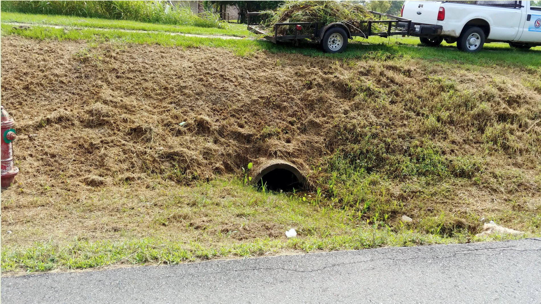
Brushy Bayou culvert on Martin Luther King Dr. near Fire Station
