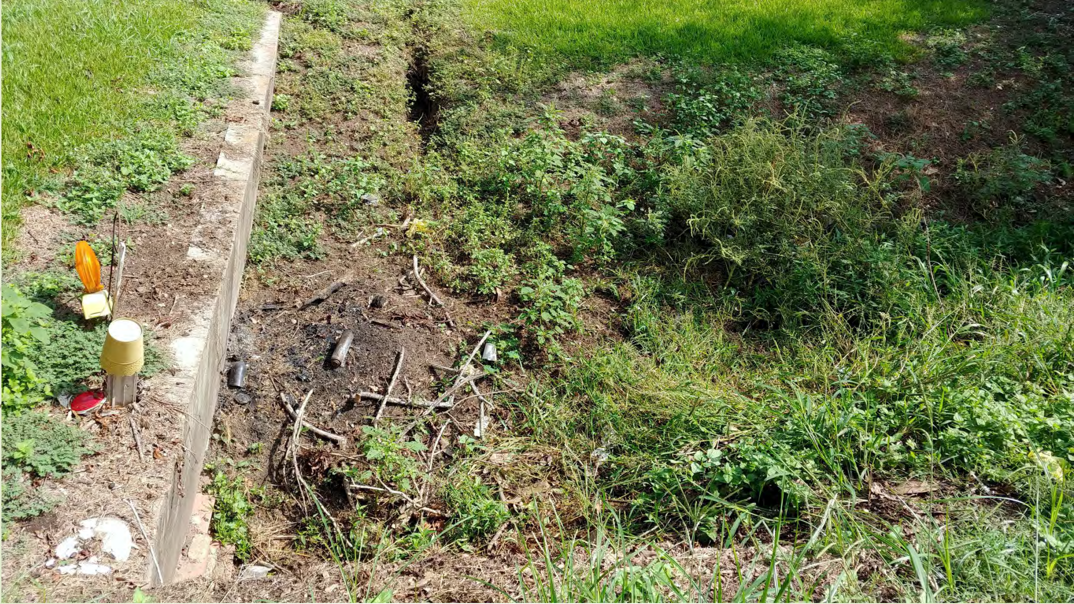
Completely blocked culvert on Riverside draining into Wilson Bayou
